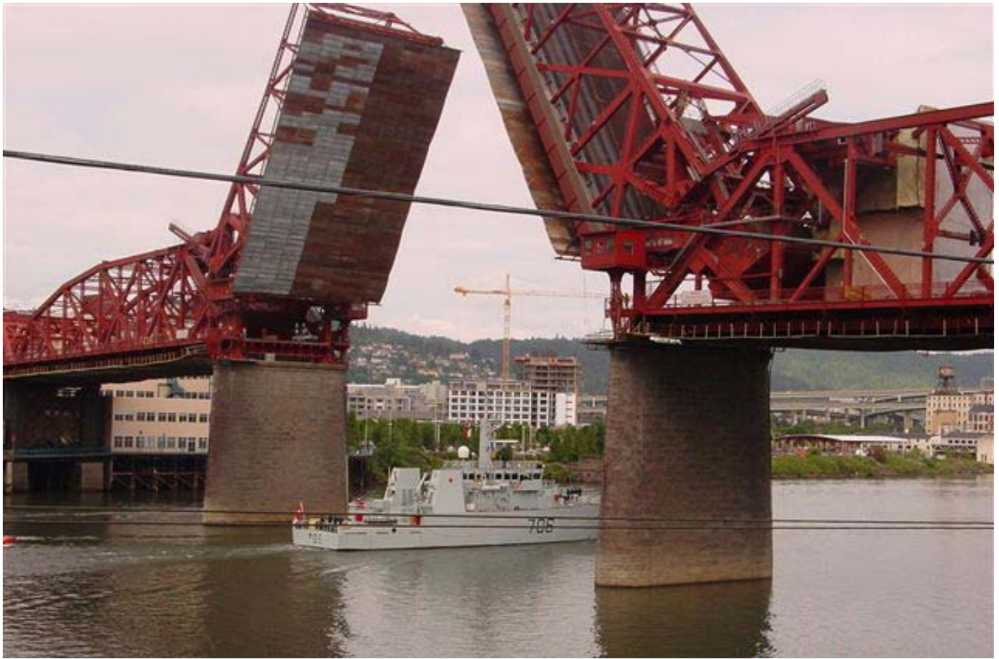
Cable Supported/Metal Deck Platform System Bascule Span Center – Truss Spans left & Right
