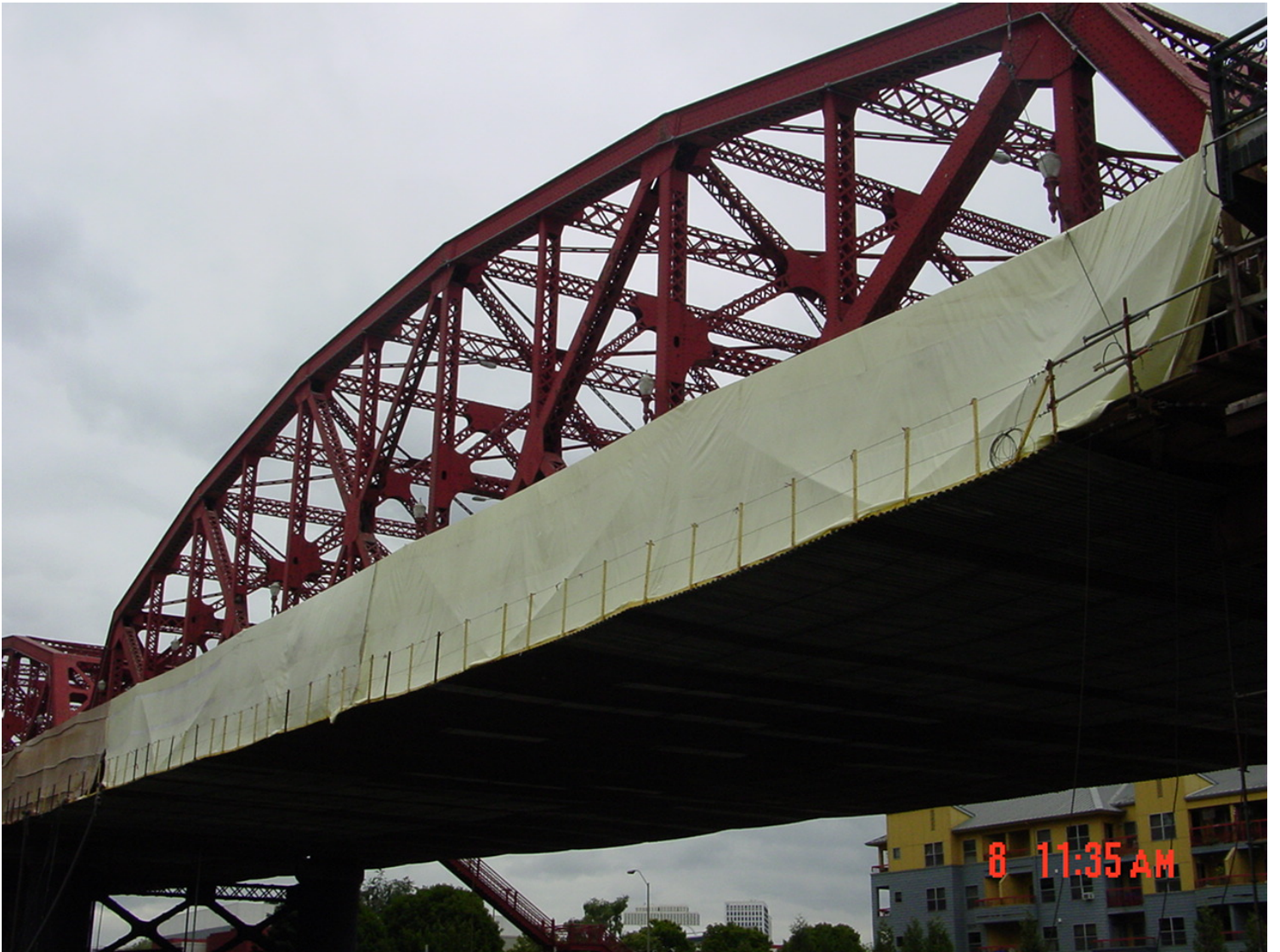
Cable Supported/Metal Deck Platform System & Containment
