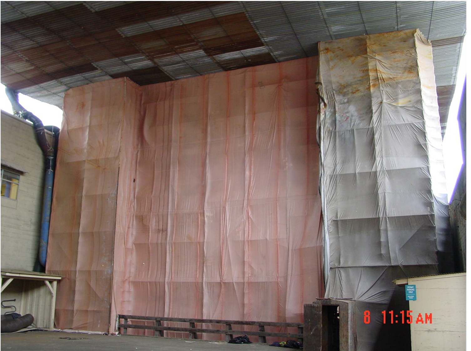
Cable Supported/Metal Deck Platform System Above Scaffold/Containment Around Bent Below
