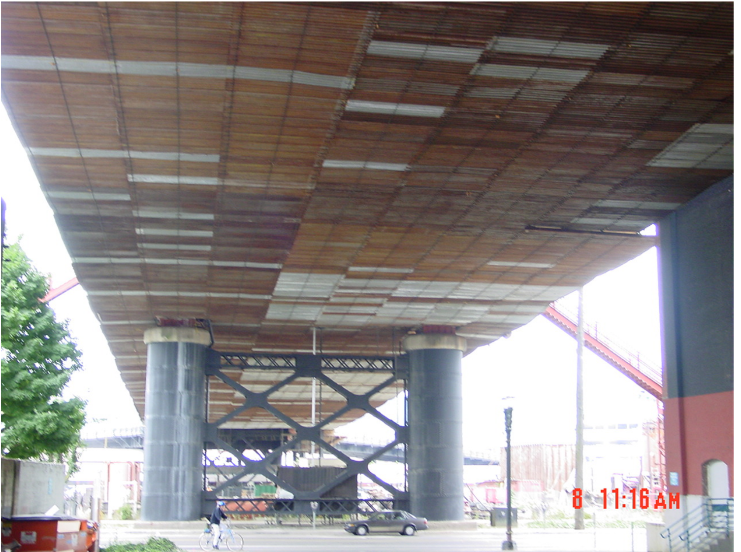
Cable Supported/Metal Deck Platform System Spans 5, 6, & 7
