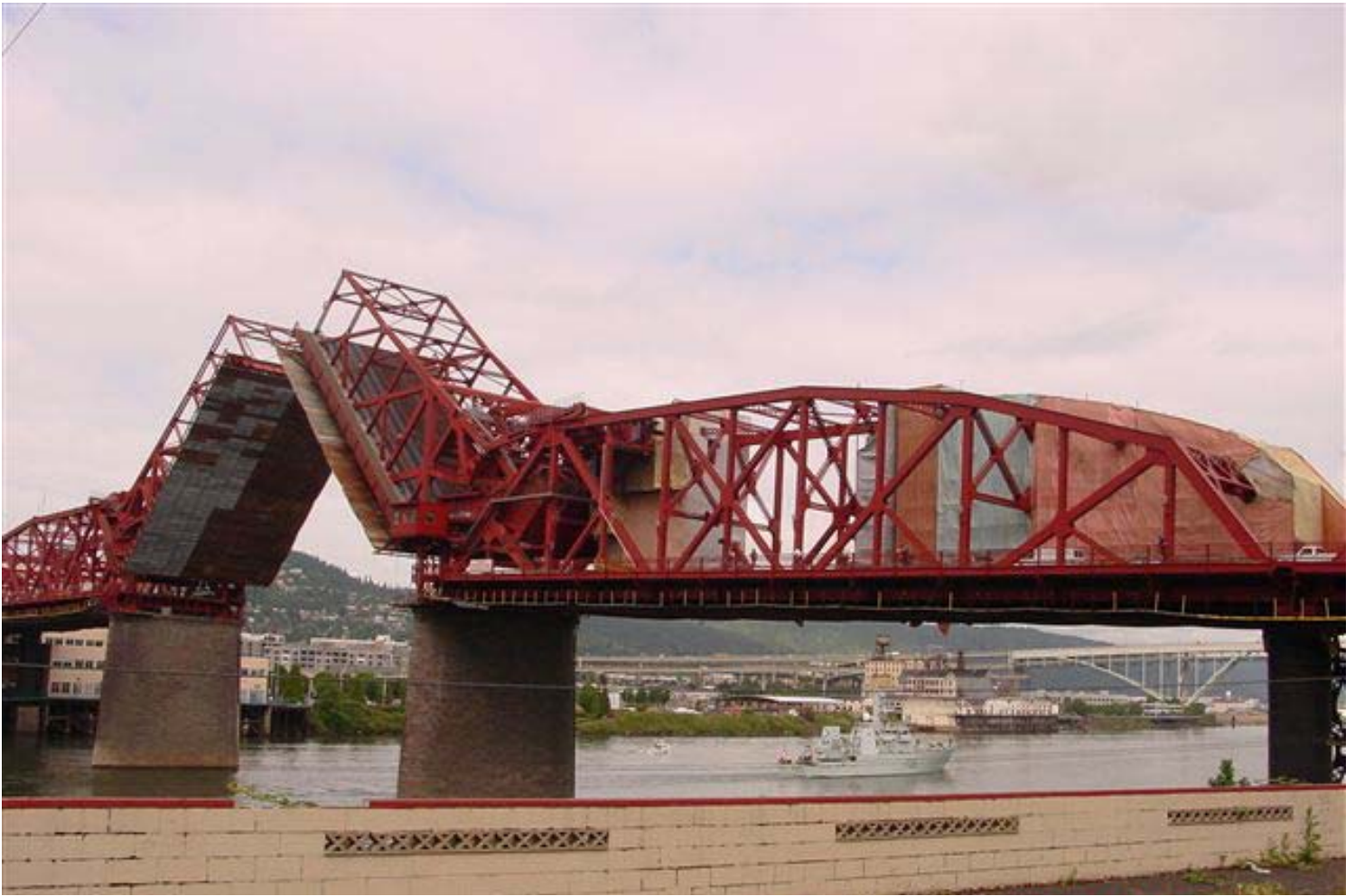
Cable Supported/Metal Deck Platform System Bascule Span Center – Truss Right W/ Containment
